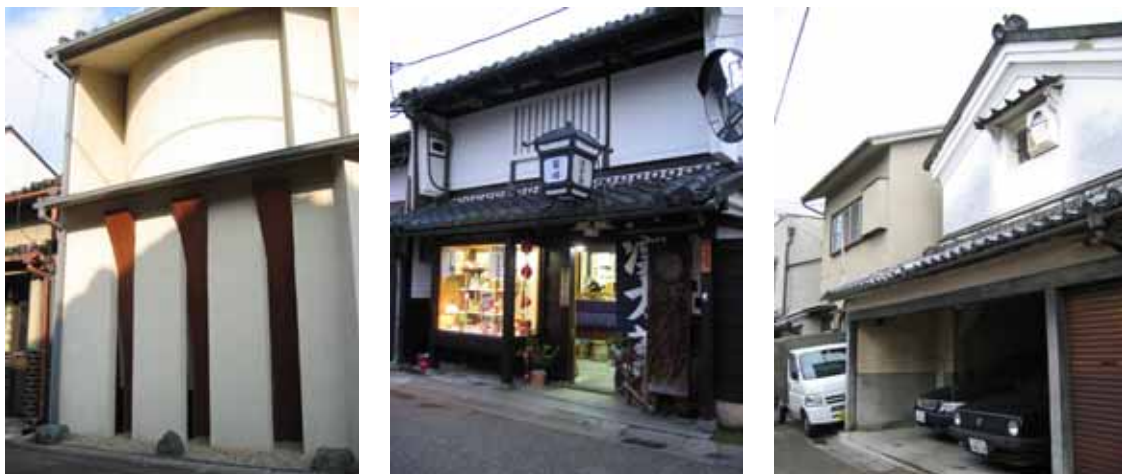
Figures 13-15: Examples of renovated traditional townhouse in the old district of Nara. Some of them are kept in originality, some are adapted to modern styles, and some are changed for comfortably uses.
